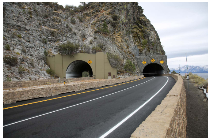
Cave Rock Tunnels—After
