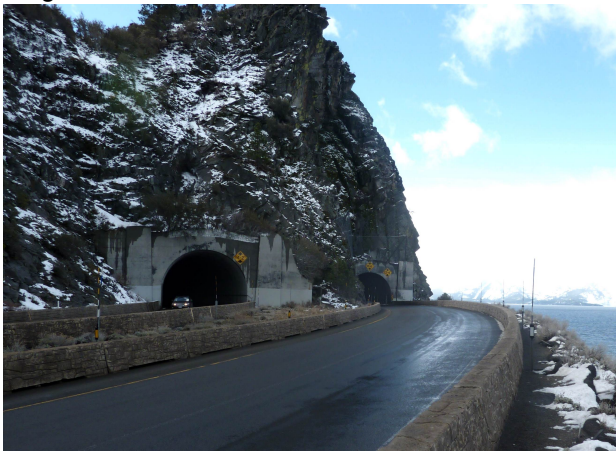
Cave Rock Tunnels—Before
